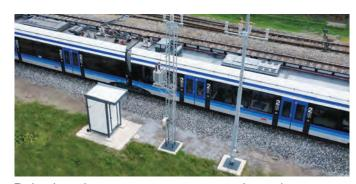
Point heating system power supply and control cabinet
