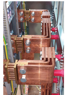
Connecting and terminal field busbars
