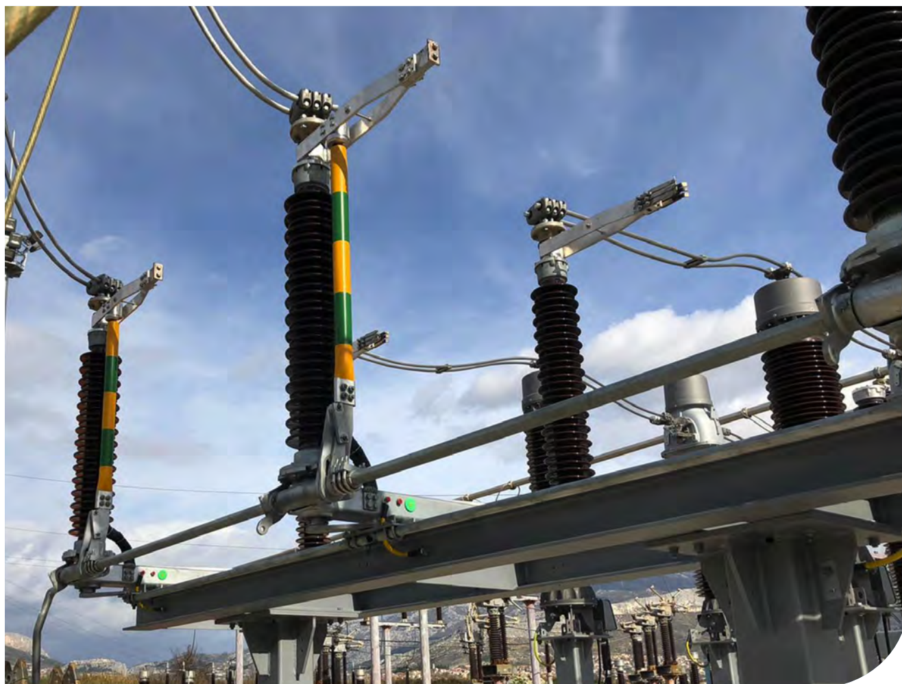
Figure 5. Central-break disconnecter series CBBe-N2 with one earthing blade installed at site (Slovakia)
