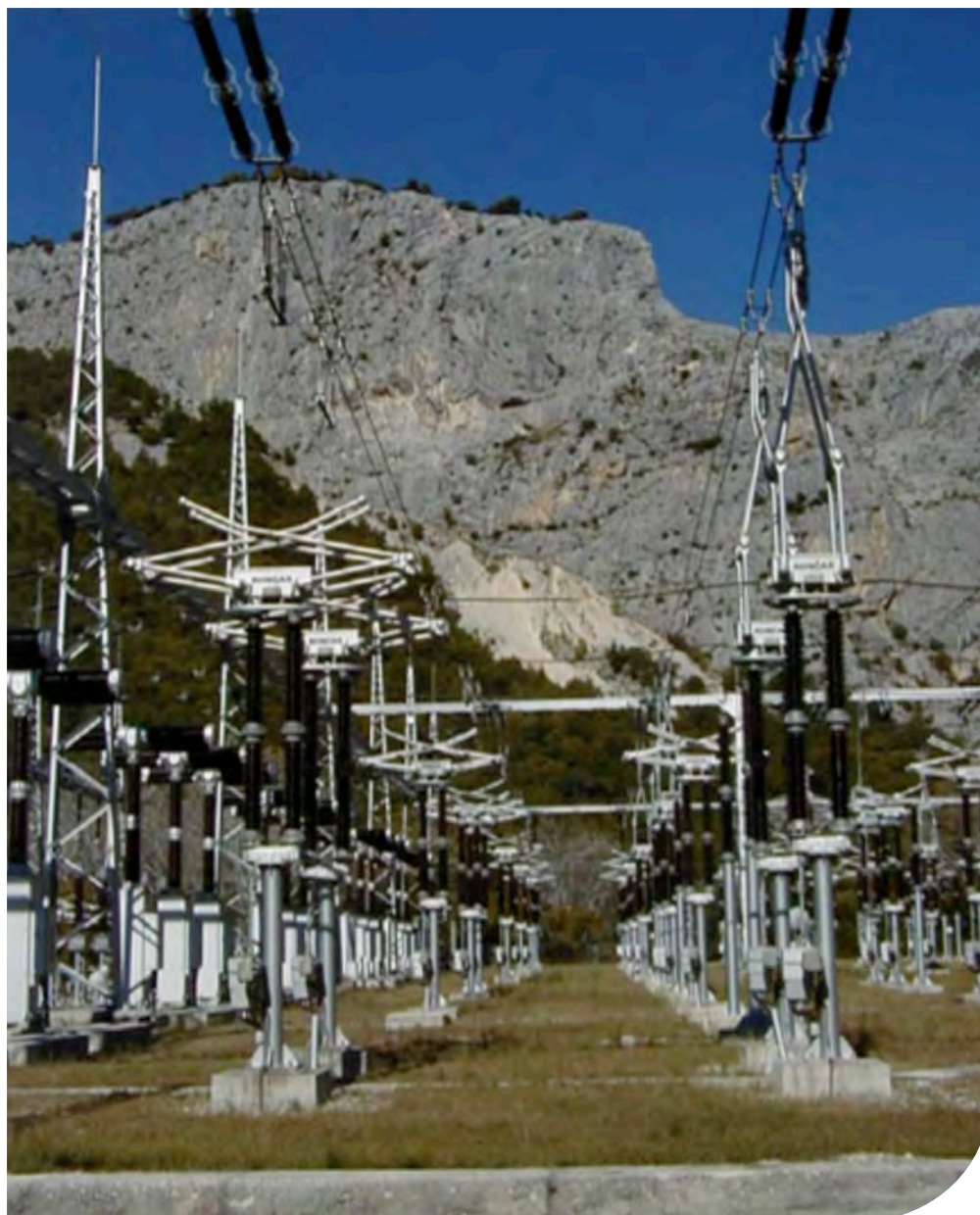
Figure 6. Pantograph disconnectors series PD in operation, hydro power plant Zakučac, Croatia
