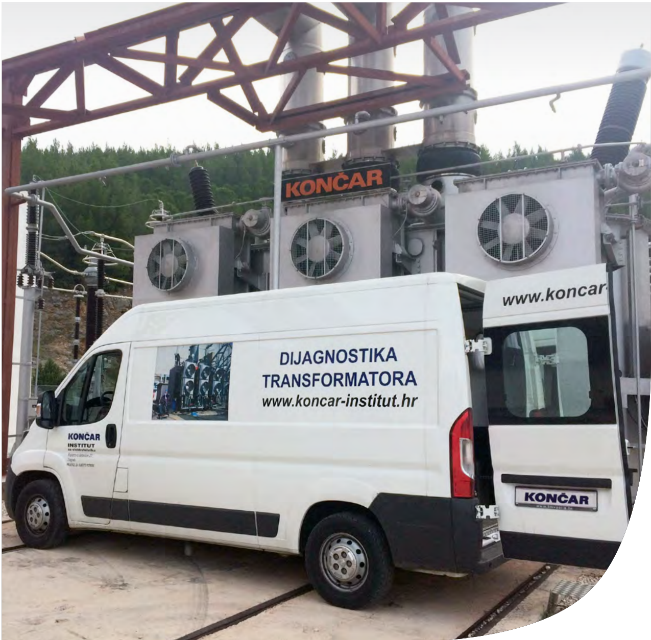
Transformer and reactor diagnostics, servicing and repairs
