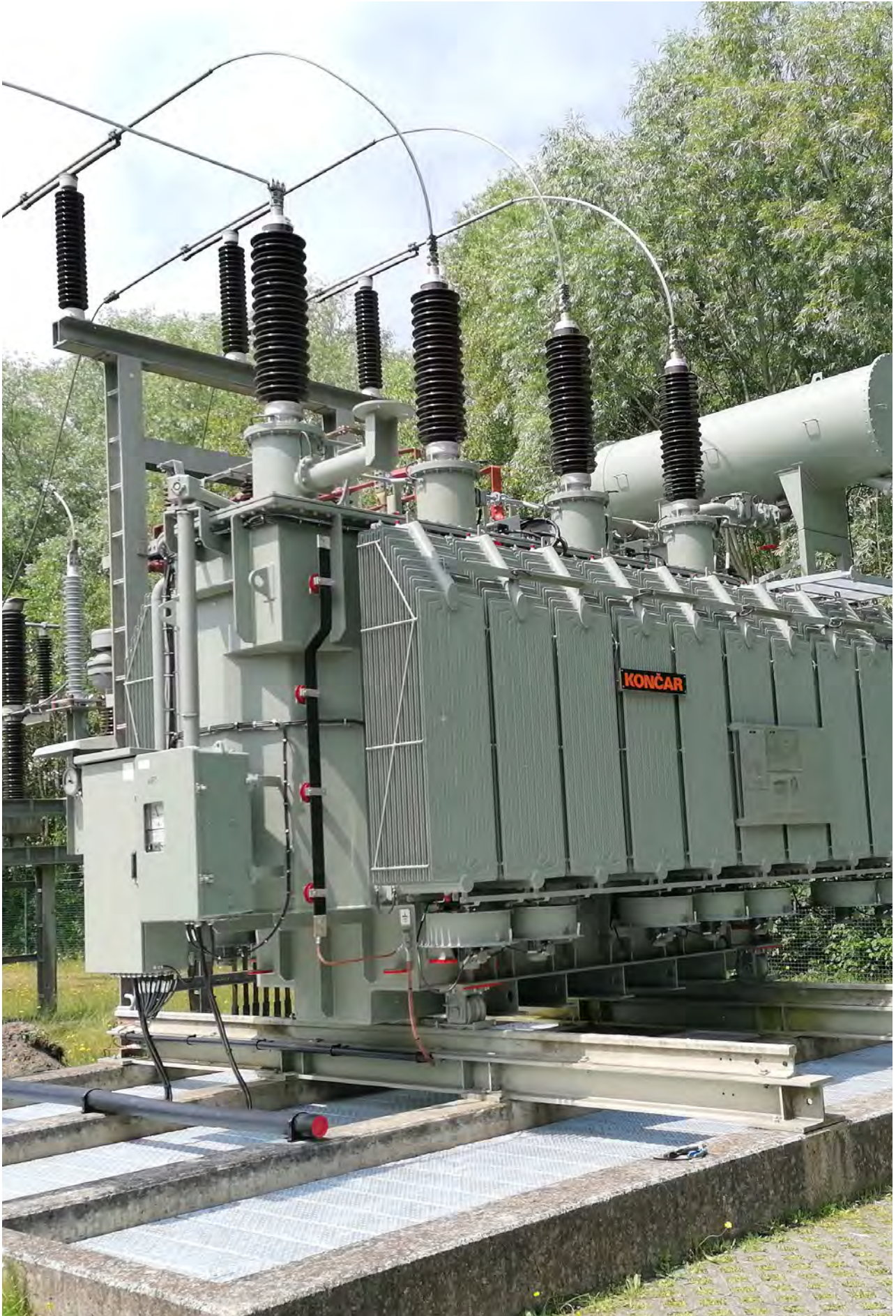
Three-phase oil immersed transformer, rated power 40 MVA
